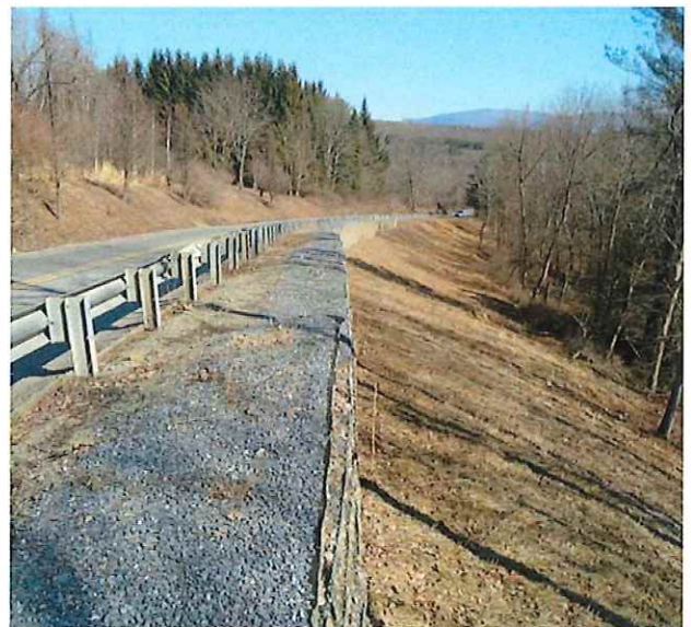
Figure 3. East, 1 Year After Completion
