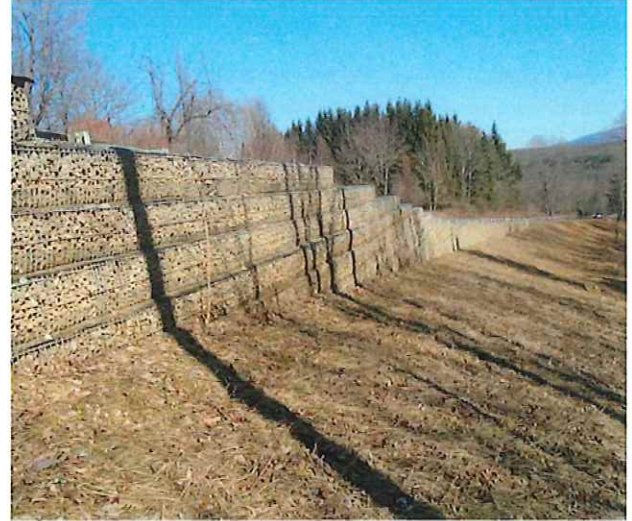
Figure 2. East, 1 Year After Completion
