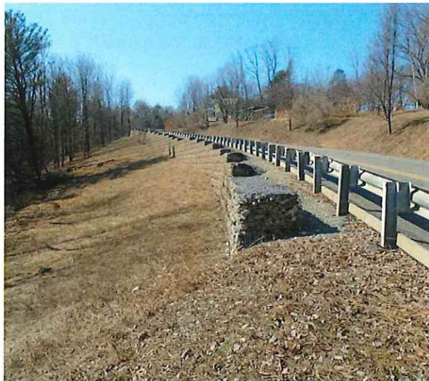
Figure 1. West, 1 Year After Completion
